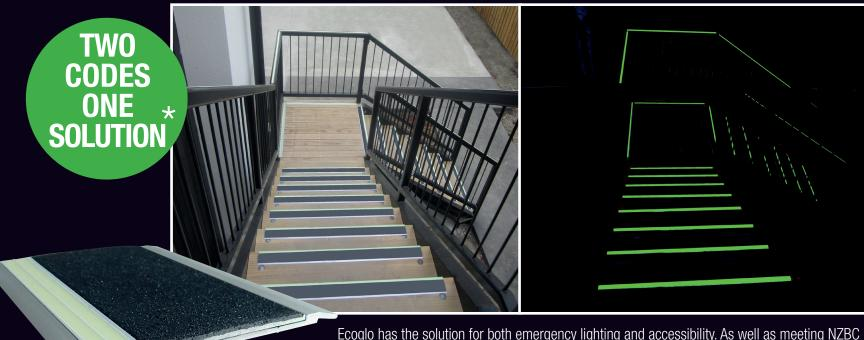
Clause D1 and AS1428.1, the F14-175 can be used to replace or enhance electrical emergency lighting in outdoor and daylit stairways. You are already installing 50mm of step edge contrast to meet D1, so use the same product to provide an emergency lighting solution.
